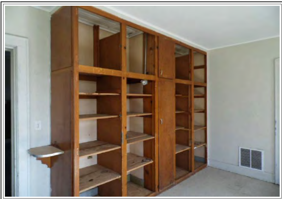
Shelves need removed and closet installed
