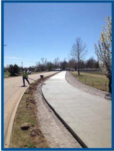
Crosslin Park pedestrian Trail: this is a 10ft wide pedestrian trail about 2.0 miles length in Crosslin Park.
