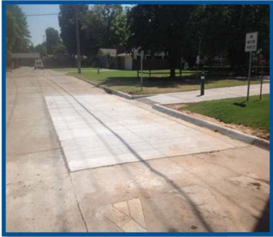
Street and Trails Repair (Parkway between Seneca and Ponca) – drainage system was implemented to alleviate the issue of standing water.
