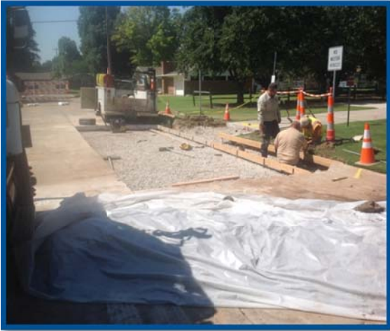
Street and Trails Repair (Parkway between Seneca and Ponca) – drainage system was implemented to alleviate the issue of standing water.
