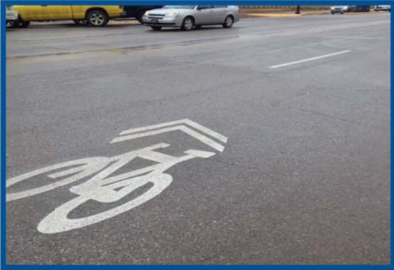
As part of City of Enid's effort to provide an alternate transportation to the residents, the project is about 4.5 miles, providing bike/motor (shared) lanes. The project consists of signage in the right-of-way and striping in the street.
