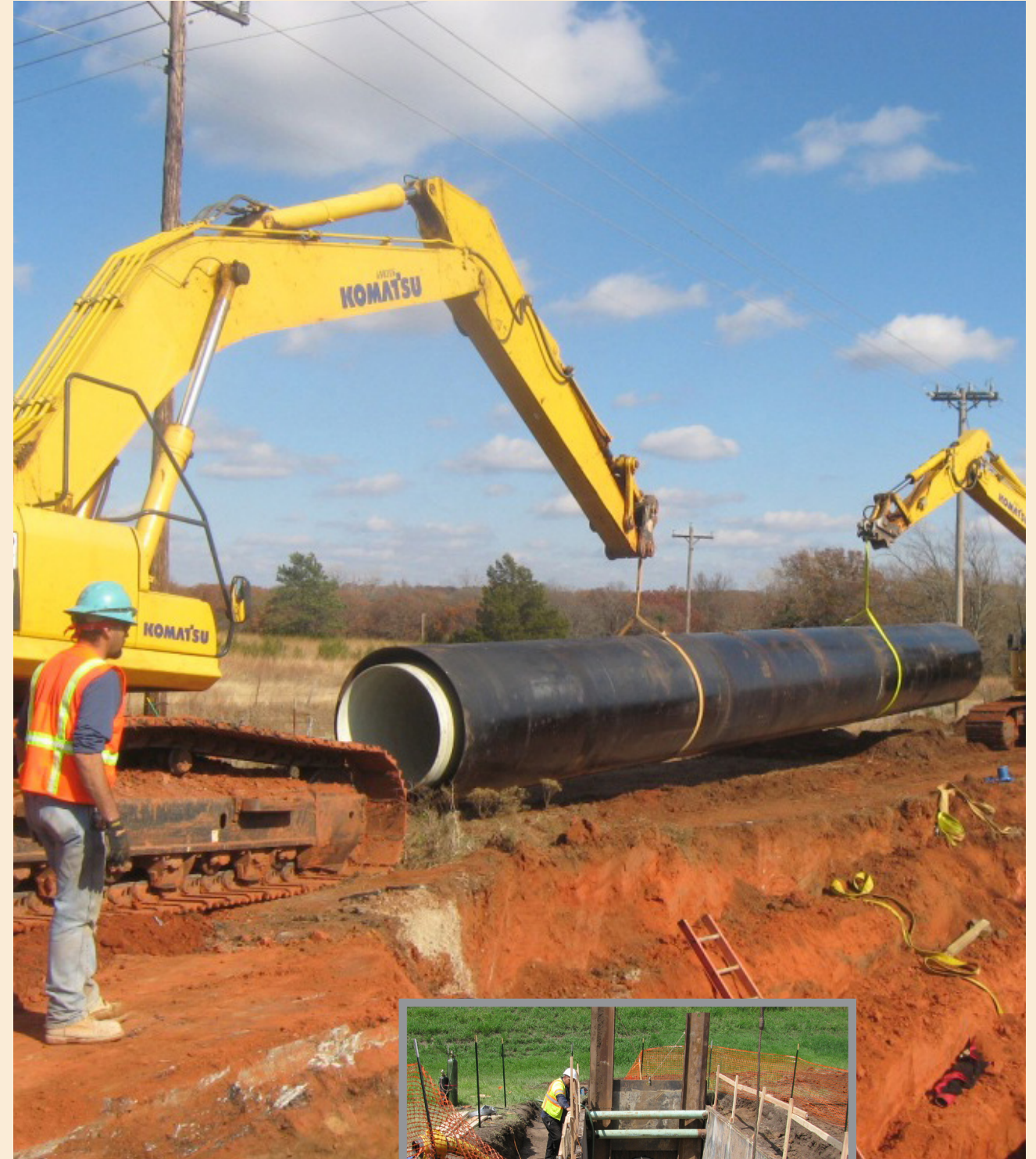
Above: Installing 60-inch casing
