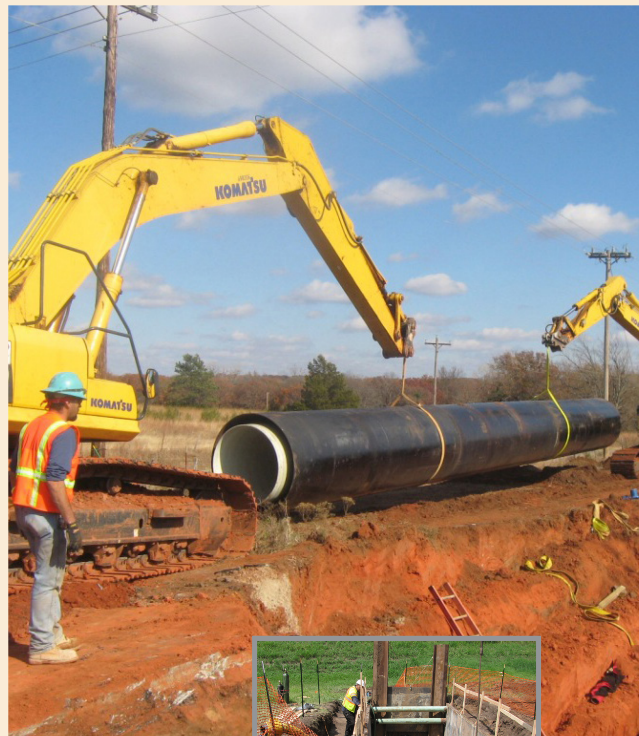
Above: Installing 60-inch casing
