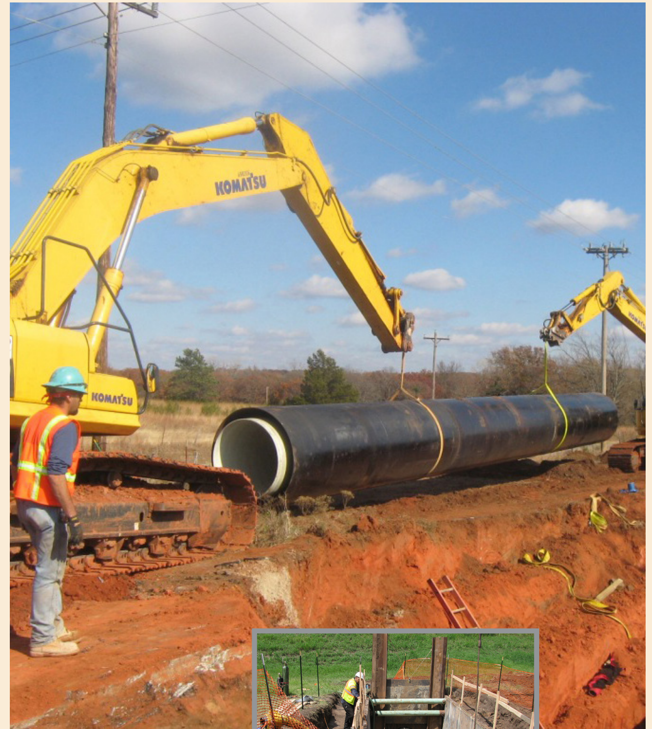
Above: Installing 60-inch casing
