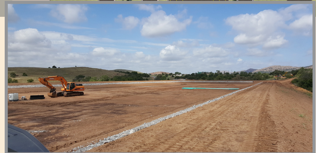
Right: Example terminal storage reservoir under construction
