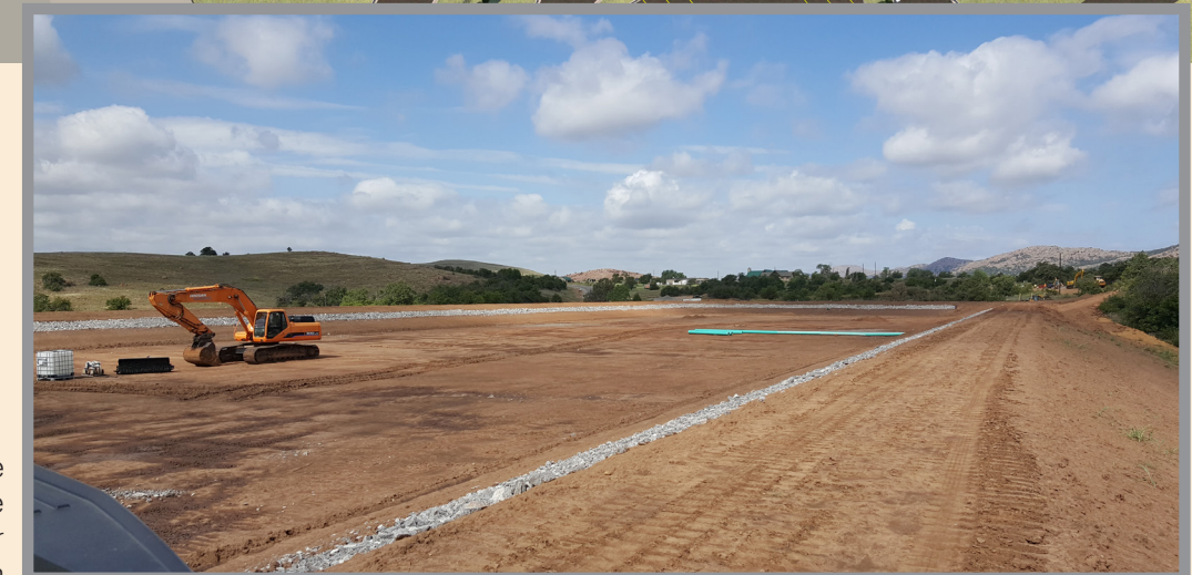
Right: Example terminal storage reservoir under construction
