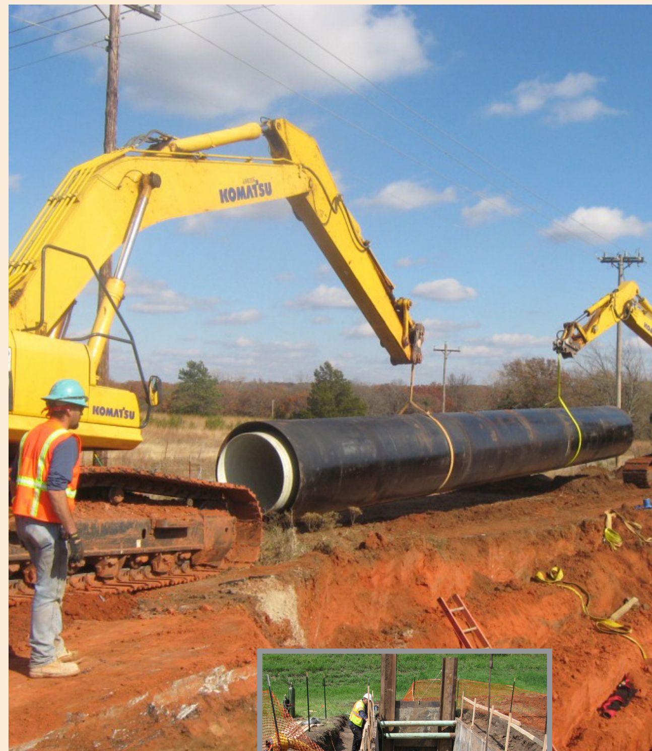
Above: Installing 60-inch casing
