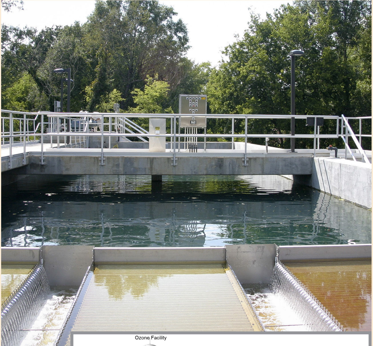
Above: Water treatment plant sedimentation basin
