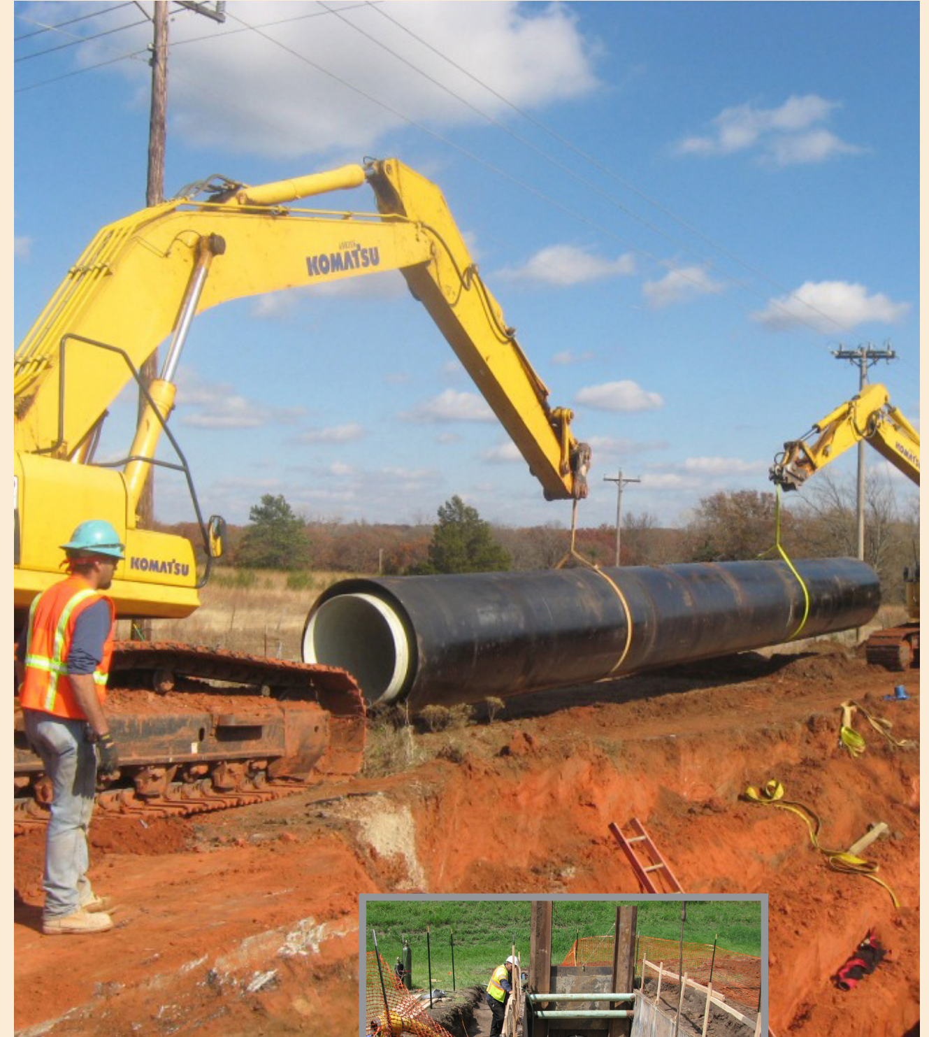
Above: Installing 60-inch casing
