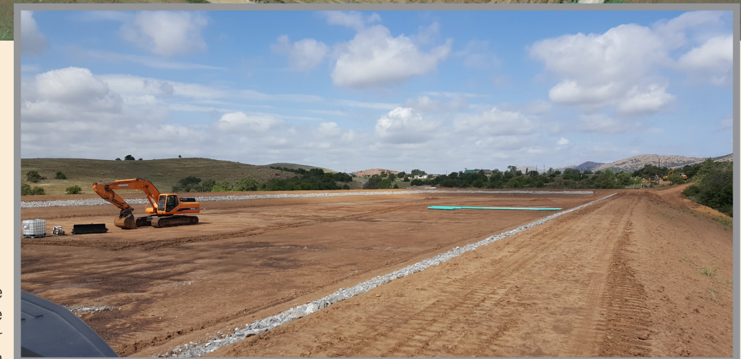
Right: Example terminal storage reservoir under construction
