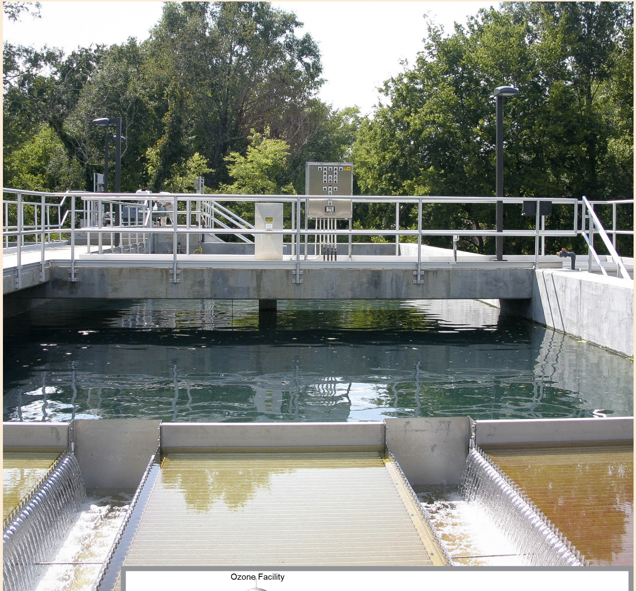
Above: Water treatment plant sedimentation basin
