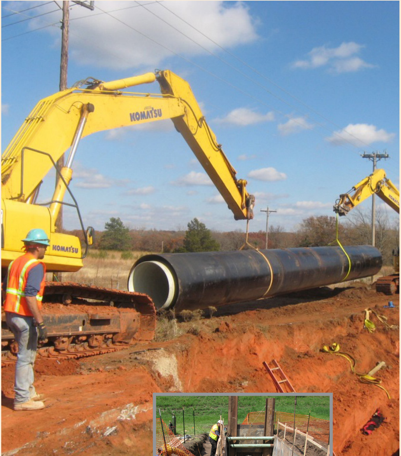
Above: Installing 60-inch casing
