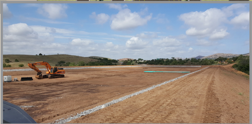
Right: Example terminal storage reservoir under construction
