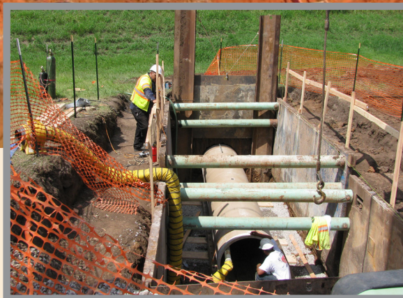
Right: Installing 48-inch pipe by bore and jack
