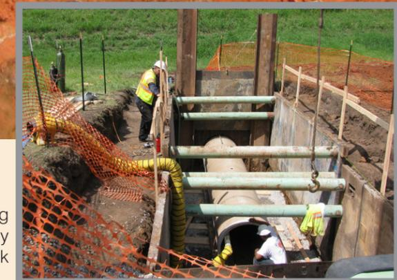
**Right:** Installing 48-inch pipe by bore and jack
