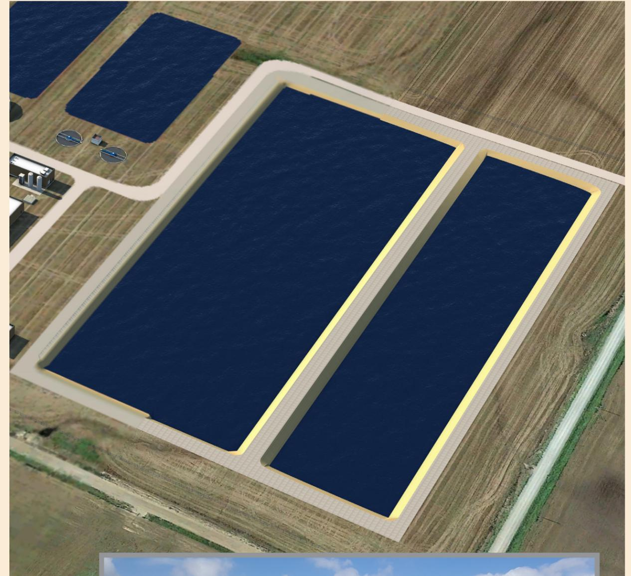
**Above:** Rendering of equalization terminal storage reservoir at water treatment plant
