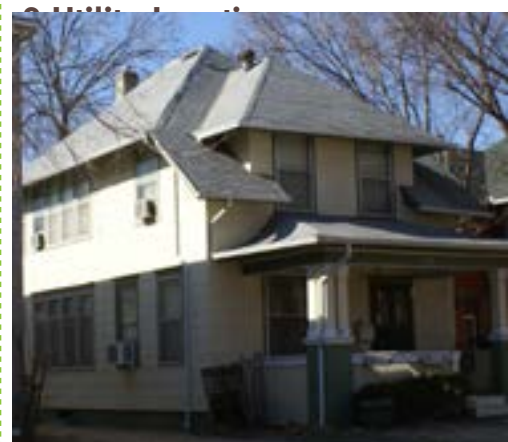
These windows units are well located on the side of the building.
