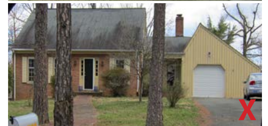
Attached garages and modern carports located in the front yard are usually not appropriate.
