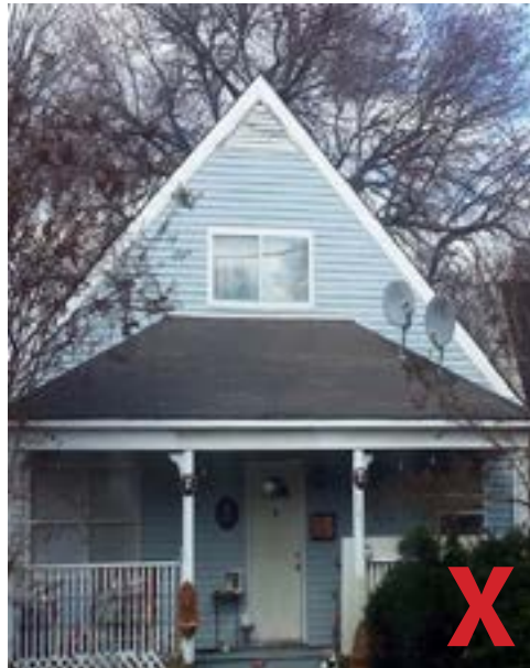
Avoid placing satellite dishes in primary facades.
