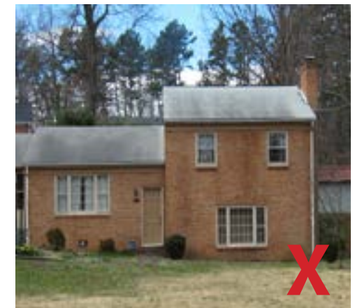
These window and door openings are not proportionate to its own structure or other homes on the street.
