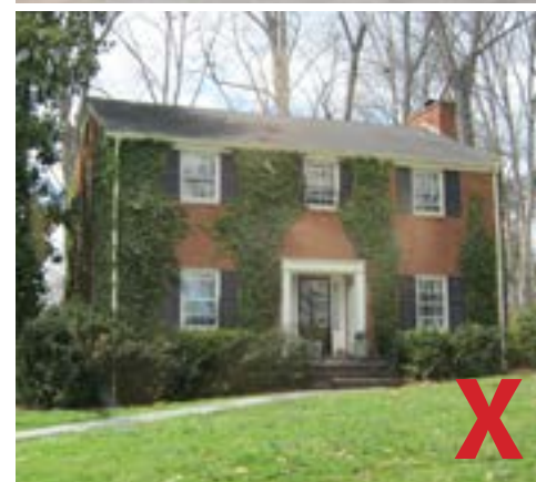
Removing all vegetation or allowing it to overgrow your building are both maintenance issues.
