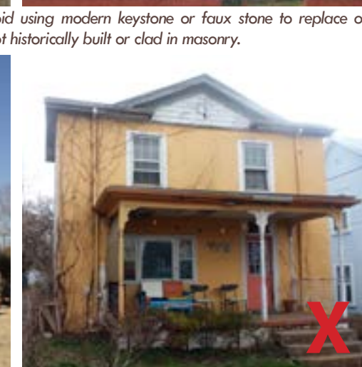
Vegetation growing on exterior walls traps moisture and is particularly detrimental to stucco.
