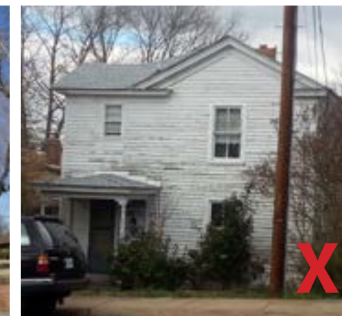
Regular painting and maintenance is the first step in preserving wood siding.
