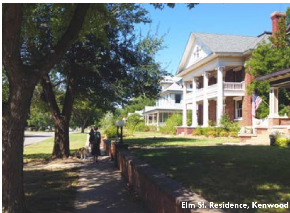
Elm St. Residence, Kenwood
