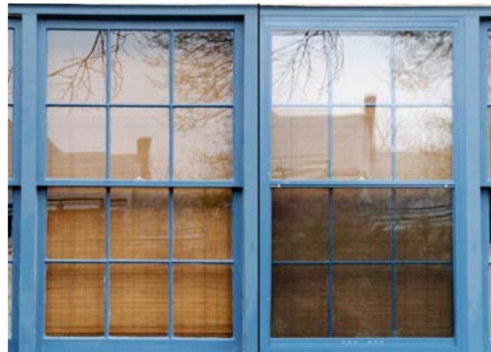
Storm windows may be installed on the exterior if the visual impact is minimal and original architectural details are not obscured.
