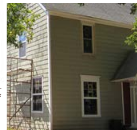
Replacement windows can be energy efficient while fitting the character and form of the original.
