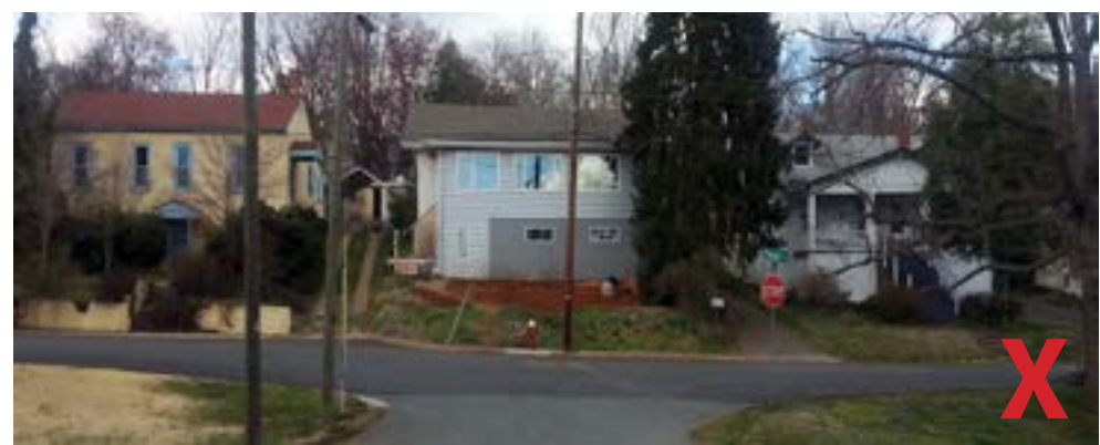
There is no consistent facade or entrance orientation on these buildings.
