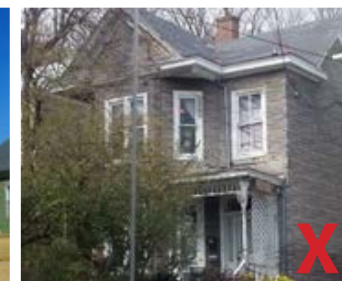
Covering wood siding with faux brick changes the character of the home and only masks water and rot issues.
