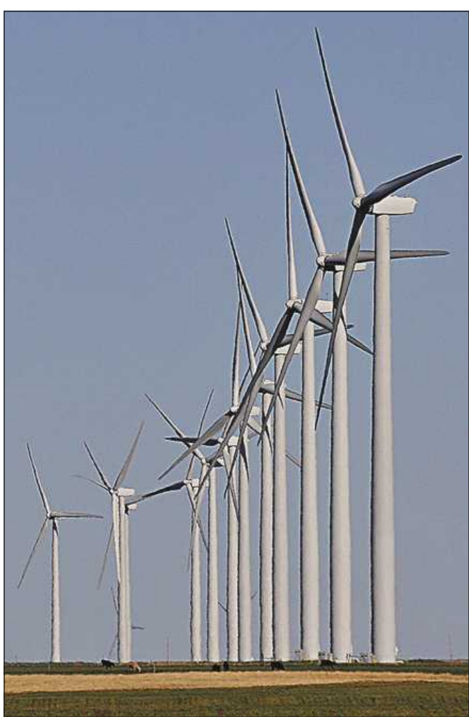
Wind turbines stand at the Chisholm View Wind Project in northern Garfield County in this March 12, 2014, file photo. (Billy Hefton / Enid News & Eagle)
