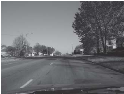
Broadway Lane corridor near E. Broadway Ave.
