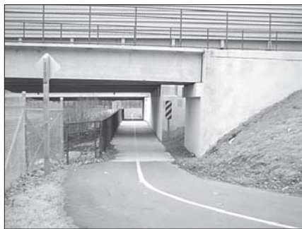
Trail Underpass with Railing
