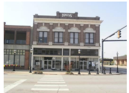
Italian Renaissance –Kress Building 129 W. Maine Street
